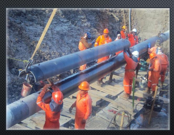
TO REPAIR LARGER AND MORE SIGNIFICANT INTEGRITY DEFICIENCIES, PREVIOUS COMPOSITE OR SPLIT SLEEVES, CURVED, ELBOWS, OR 'T' SECTIONS OF PIPING, MAJOR DENTS, LEAKS, ILLEGAL TAPS OR UNIQUE CONDITIONS
