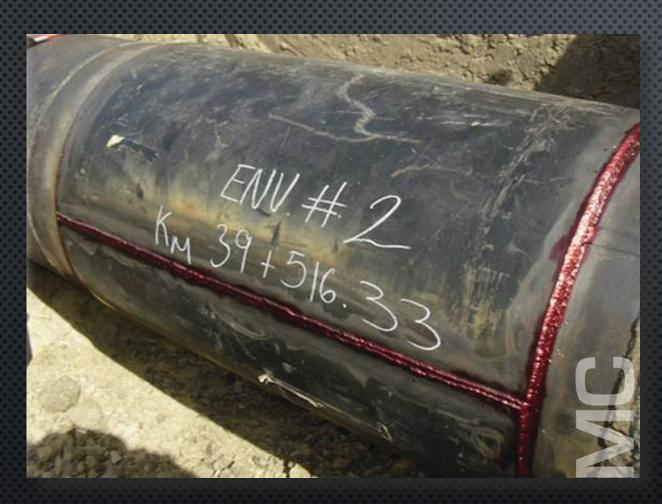
INSTALLED WITH LONGITUDINAL AND CIRCUMFERENTIAL WELD APPLICATION TO THE PIPELINE
