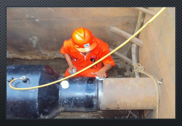
CUSTOM MADE WITH CONCENTRIC REDUCTIONS AND PRESSURE FILLED TO ELIMINATE VOID SPACE
